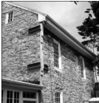
Renovations were undertaken by the Civic Club in the 1930s, 1960s, and 1970s. By 2002, bowing of the Queen Street wall was putting pressure on window frames creating fissures allowing rainwater to infiltrate the building. A project to address the root causes of the problems - funded entirely with private money - was undertaken by the Club.
