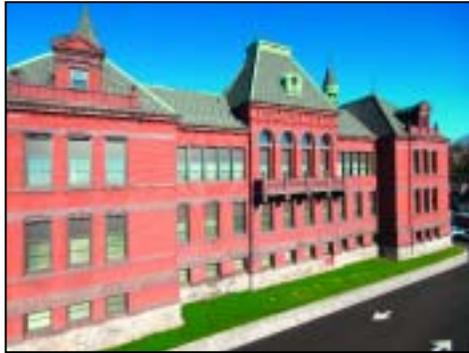
in-kind repairs to sandstone detailing. The slate roofs were replaced with new material that replicated the appearance of the deteriorated slate, and roof features such as cupolas and dormers were repaired. Although the budget did not allow for the replacement of existing replacement windows with historically appropriate sashes, the only notable exterior alteration was the sensitively located and designed entrance to the indoor parking garage.
