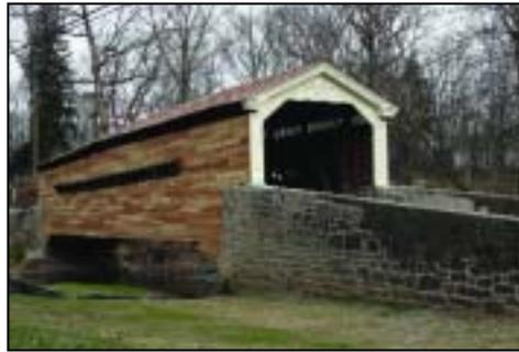
siding and trim, floor planks, decking, and curbs, were all removed and replaced in kind, as were selected wood framing members, including roof rafters, ceiling joists, knee bracing and siding studs. A clear fire retardant wood preservative was applied to the structure, and the portals were repainted.
