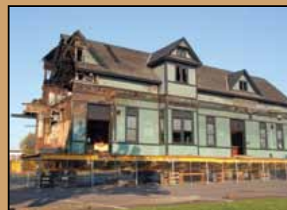
Partially demolished Depot on cribbing awaiting its new foundation. Cover photo of Pennsylvania At Risk in 2010.
