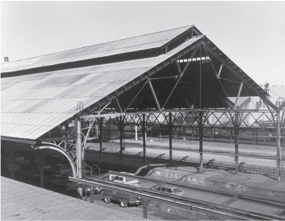
The Harrisburg Trainsheds are recognized by the National Park Service as one of Pennsylvania's National Historic Landmarks because of their distinctive Fink truss system.
