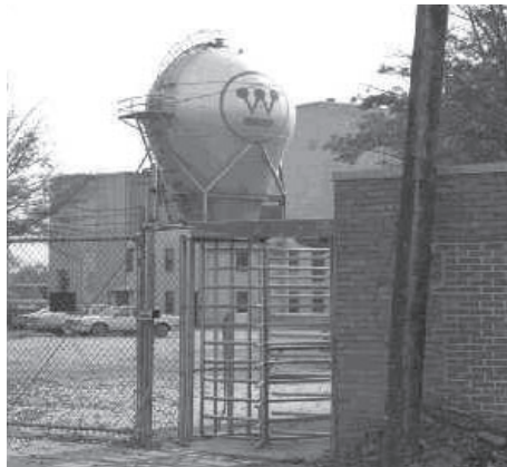
The 1937 five million volt van de Graaf Atom Smasher Generator represents the first large-scale program in nuclear physics established in private industry. Photo Source: IEEE History Center
