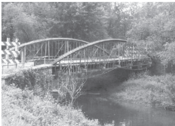
Henszey's Bridge over Ontelaunee Creek, a 1869 wrought-iron bowstring truss bridge. Photo courtesy of Central Pennsylvania College
