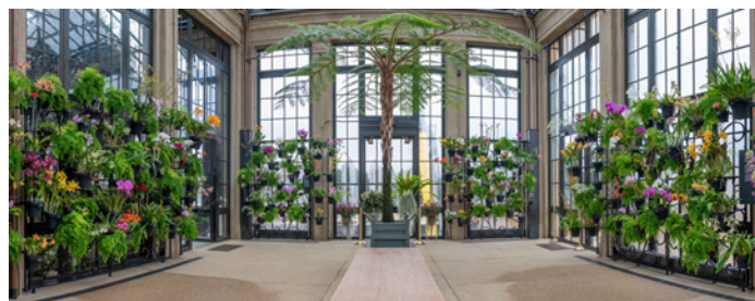
Top: The completed exterior restoration of the Orchid House is shown facing northeast. Exterior site work continues as part of the larger Longwood Reimagined project. Bottom: Overview of the restored windows, doors, frames, Earley concrete, and orchid displays on each wall.
