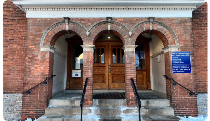
Sunday school building, main entrance. Credit: Blake Gifford
