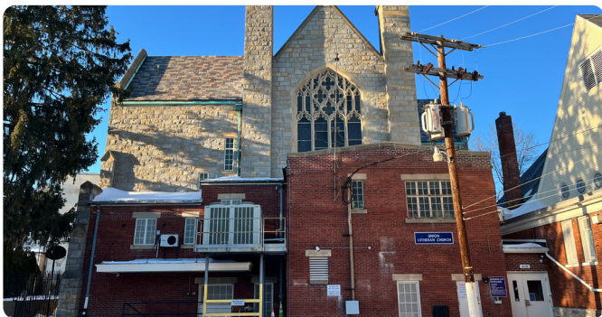
Sanctuary building, south (rear) facade. Credit: Blake Gifford
