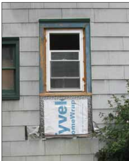
Because this window replacement is changing the size of the window opening, it is not appropriate.
