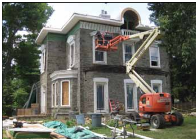
The windows on this building are being replaced with windows of an inappropriate type, pane configuration and possibly material.
