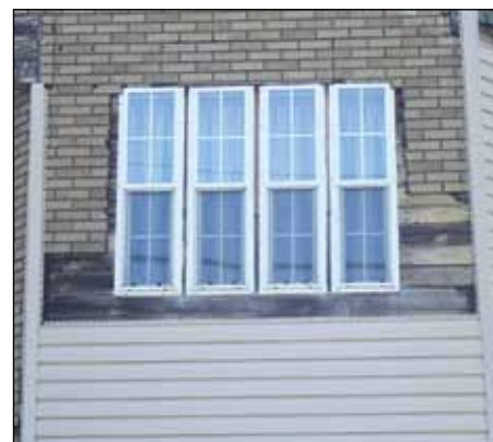
This window replacement used windows of the wrong size, shape and pane configuration for the window opening, and failed to maintain the existing trim.
