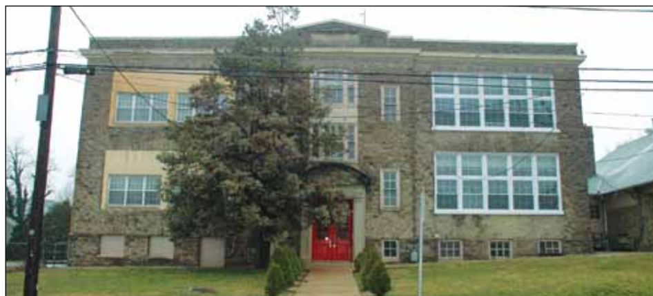
This historic school building is in its second cycle of window replacement. Those in the center bay and basement appear to be original. The windows on the left were replaced inappropriately with smaller windows that required alteration of the original window opening. The windows on the right, which are replacing earlier replacements, are restoring the size of the window opening and approximating the original pane configuration.
