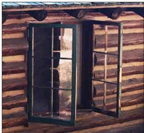
These historic windows have full screens inside the casements, which are hinged to open easily to facilitate window operation.
