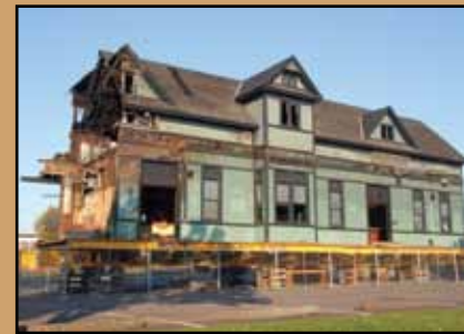
Partially demolished Depot on cribbing awaiting its new foundation. Cover photo of Pennsylvania At Risk in 2010.
