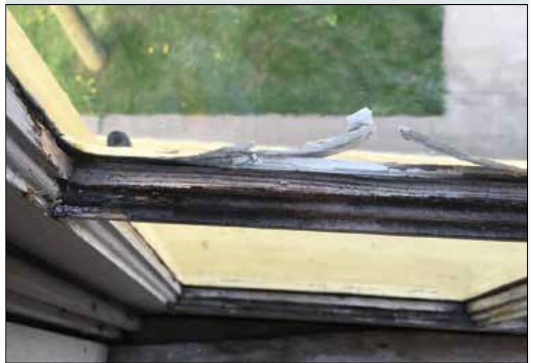
The staining on the muntin, rail and sill of this window are the result of condensation.
