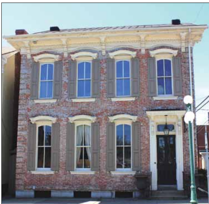
Can you see the storm windows on this historic house? The left three windows on the second story have exterior storm windows, while the others do not.
