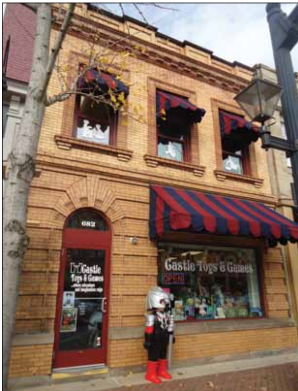
Awnings are a historic method of shading that is still a viable way to reduce solar gain today.
