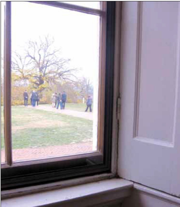
The staining on the muntin, rail and sill of this window are the result of condensation.
