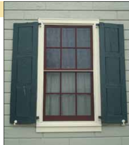
This aluminum-clad replacement window is well-suited to this historic building.
