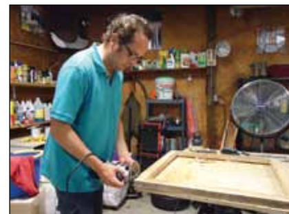
As part of a comprehensive restoration and energy upgrade, a homeowner routs his historic window sash to insert weather stripping.
