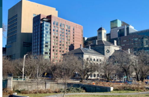
Charles Street Jail exterior
