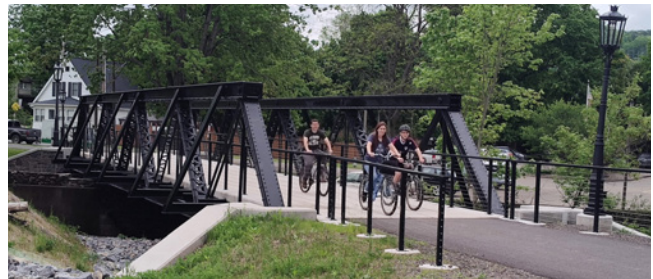
Upper left: View of the Howellville Truss being prepared for transportation to Tioga County during the removal/relocation process (Photo credit: Wilson Consulting Group) Upper right: End view of the completed bridge. The bridge width was reduced from 21.3' to 15' (center-to-center). (Photo credit: Wilson Consulting Group) Bottom right: View of the bridge being used by bicyclists (Photo credit: Wilson Consulting Group)
